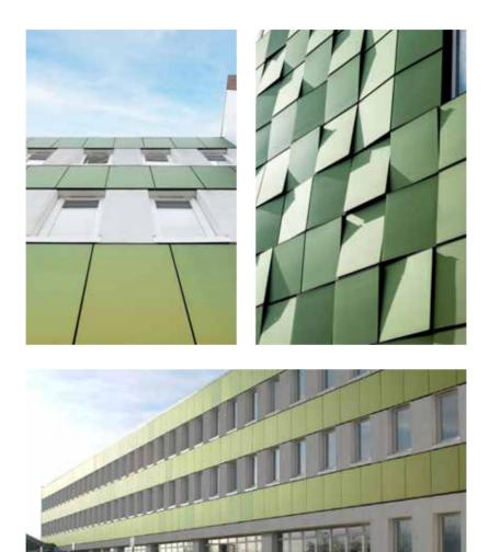
solar panels: planar and tilted in four directions
